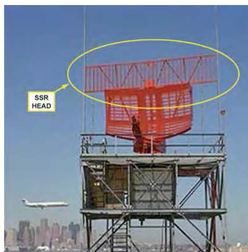
Figure 20.1 A secondary surveillance radar head, on top of a PSR head.
