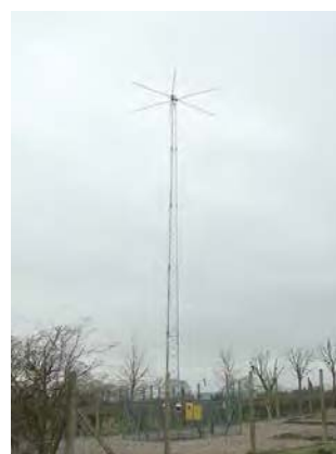
Figure 16.2b A Non - Directional Beacon (Photo courtesy of Trevor Diamond www.trevord.com ).
