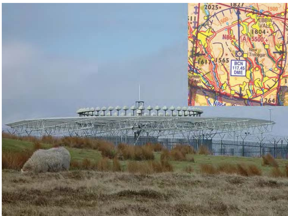
Figure 17.16 The Brecon VOR/DME and its location on the 'half-mile' chart. (Photo by kind permission of Trevor Diamond –www.trevord.com).
